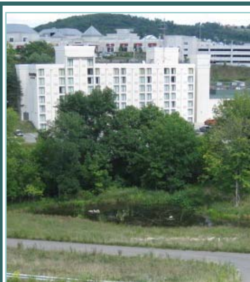
At Tanger Outlets: Detention Pond to help control stormwater runoff
